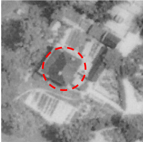
Fig 27. Aerial Photo of the SSQ in 1949 shows the roof of the Main Building as hipped pitch roof. (Source: Survey and Mapping Office, Hong Kong)
