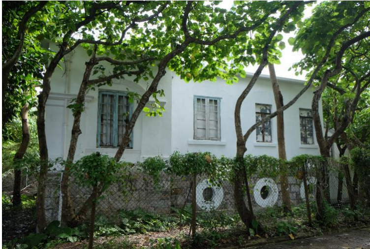
Fig 53. View of the SSQ after repair works, 2016 (Source: Photo taken by Betty Tay)
