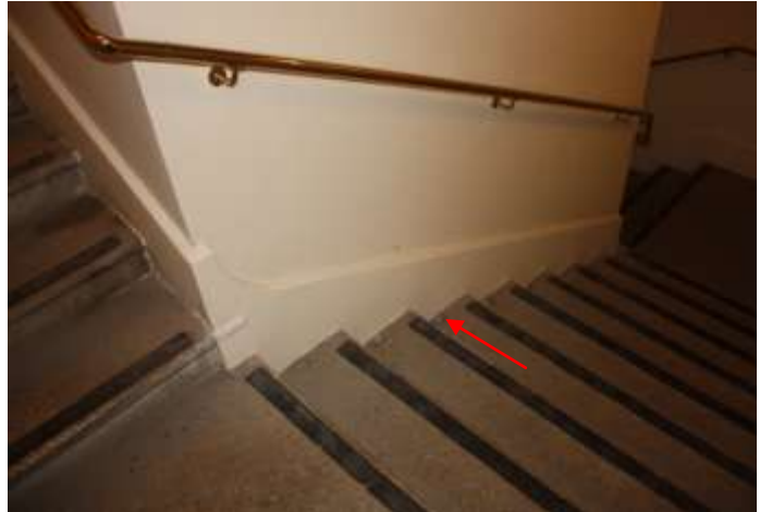
Fig.69 (left) and Fig. 70 (right) The preserved original granite staircase including the exposed granite steps and the footings with traces of original footing of the handrails (pointed).
