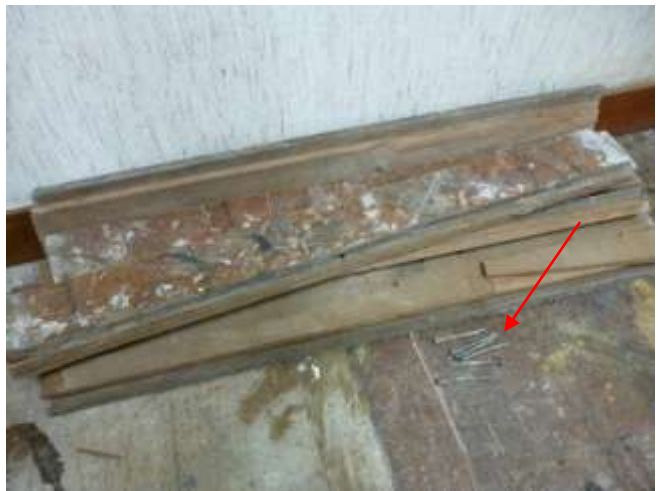
Fig. 73 (left) Pictures showing a room with original timber strip flooring. The floor was damaged by trunk work (pointed)
