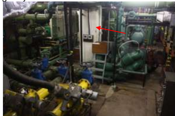
Fig. 37 (Right) The general view of the existing basement used as the plant room. A load bearing column constructed at the centre supporting the entire floor
