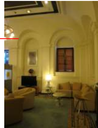
The Dining Room with original arch and pilaster moulding features still existing in 2/F
