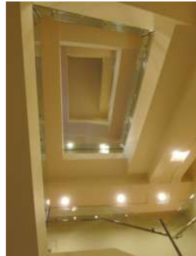
Fig. 71 (left) and Fig. 72 (right) One of the typical layout of the two reconstructed staircases done in 1985 conversion work. The staircase is constructed with concrete with glass panels balustrades spiraling around the central well to 2/F.
