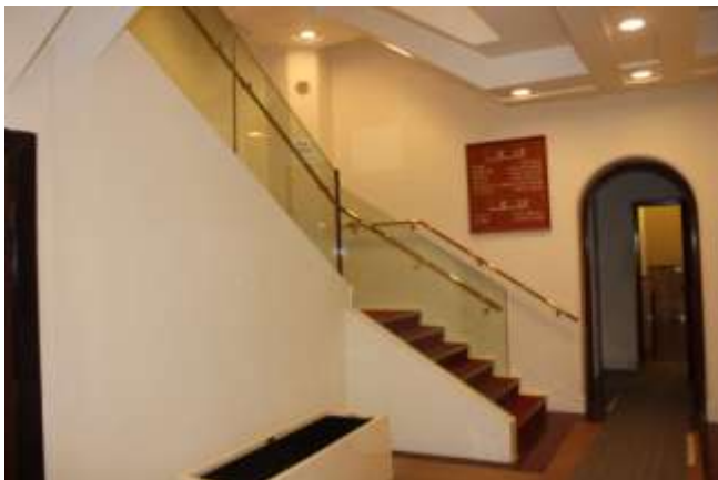
Fig. 71 (left) and Fig. 72 (right) One of the typical layout of the two reconstructed staircases done in 1985 conversion work. The staircase is constructed with concrete with glass panels balustrades spiraling around the central well to 2/F.
