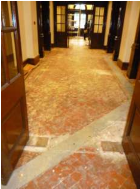
Fig. 78 (left) and Fig. 79 (right) Pictures showing the discovered original floor tiles (Fig. 78) with its detailed patterns (Fig. 79) found in the corridor areas located in 1/F and G/F respectively.
