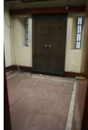
The prisoners' receiving entrance area with terrazzo floor finish
