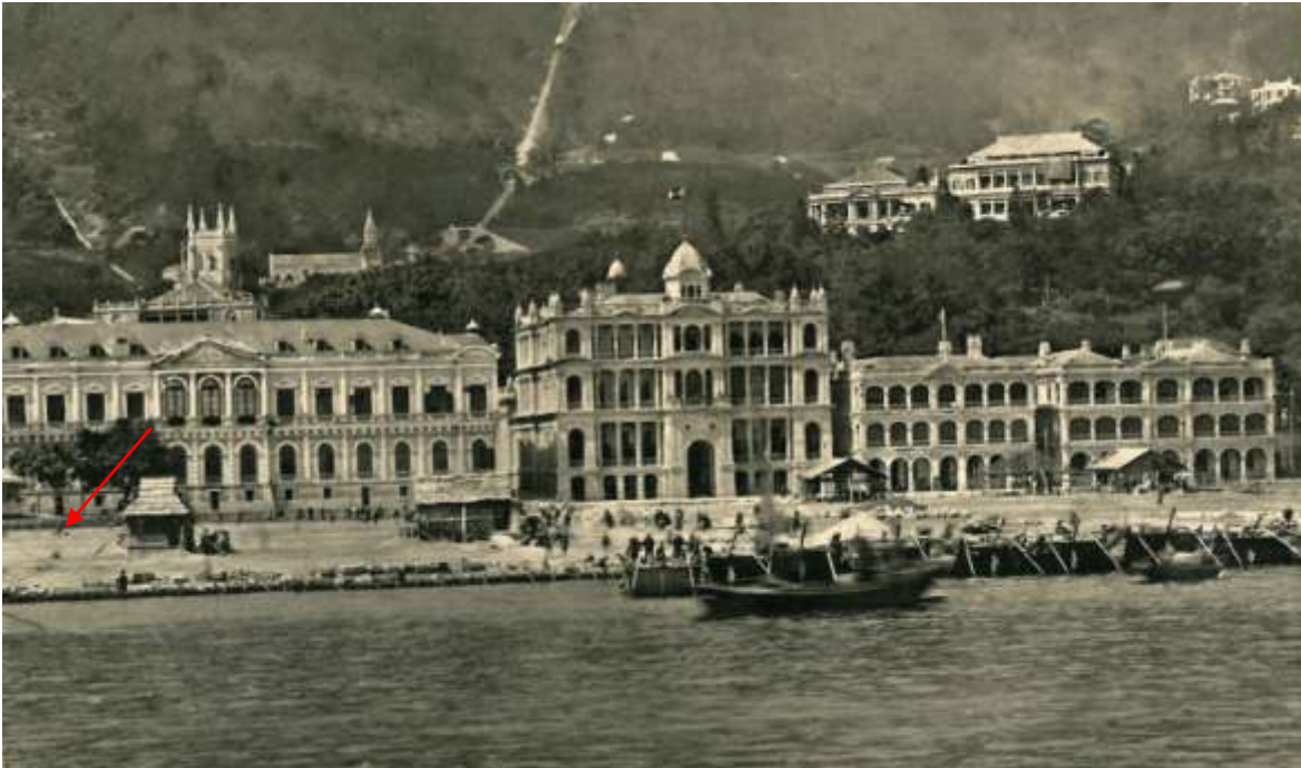
Fig. 5 The new praya of Central nearly completed from the Scheme. The first structure being erected in this new land was the Queen's Statue being in place in 1896. The site of Supreme Court Building was planned to occupy the site left of the straw shed (pointed) just in front of the old City Hall (left building). The middle building was the 2 nd HSBC Building; Photo taken before 1896. (Source: Once Upon A Time – Hong Kong, FormAsia, 1 st publishing, 2011)
