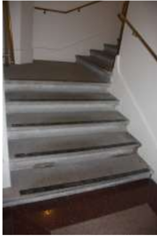
Fig.69 (left) and Fig. 70 (right) The preserved original granite staircase including the exposed granite steps and the footings with traces of original footing of the handrails (pointed).
