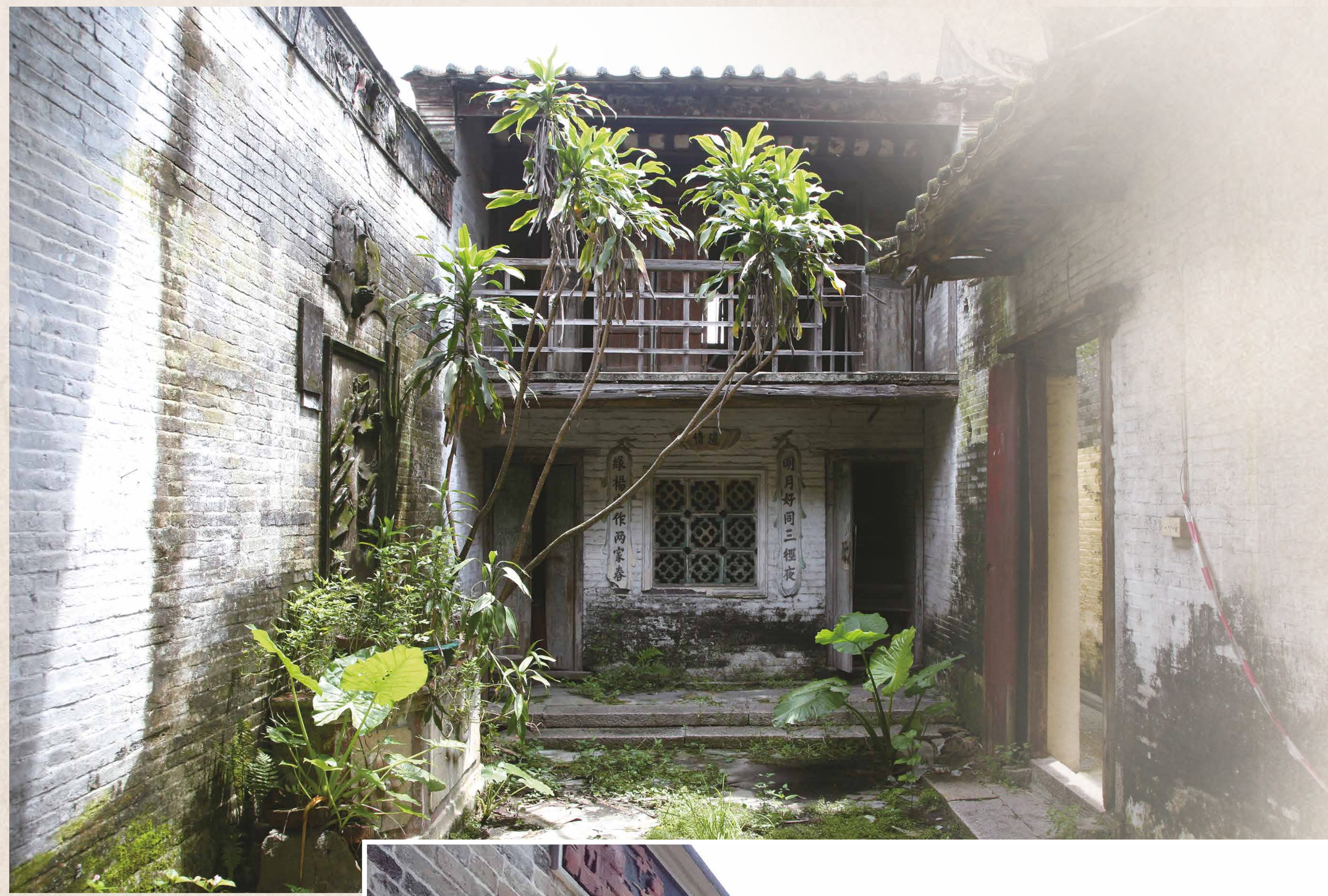
修復前的禮賓樓倒座及天井 The front block and open courtyard of Guesthouse before restoration
