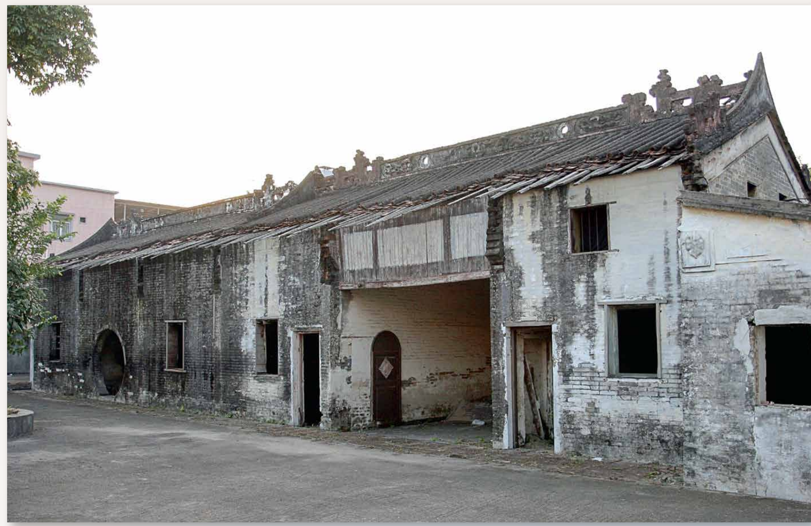
修復前的友恭學校 Yau Kung School before restoration
