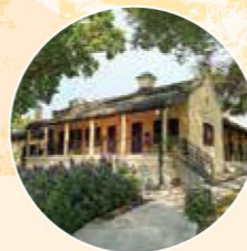
舊大埔警署 Old Tai Po Police Station
