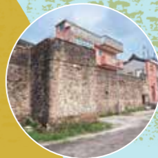
泰亨灰沙圍圍牆 Enclosing walls of Fui Sha Wai, Tai Hang
