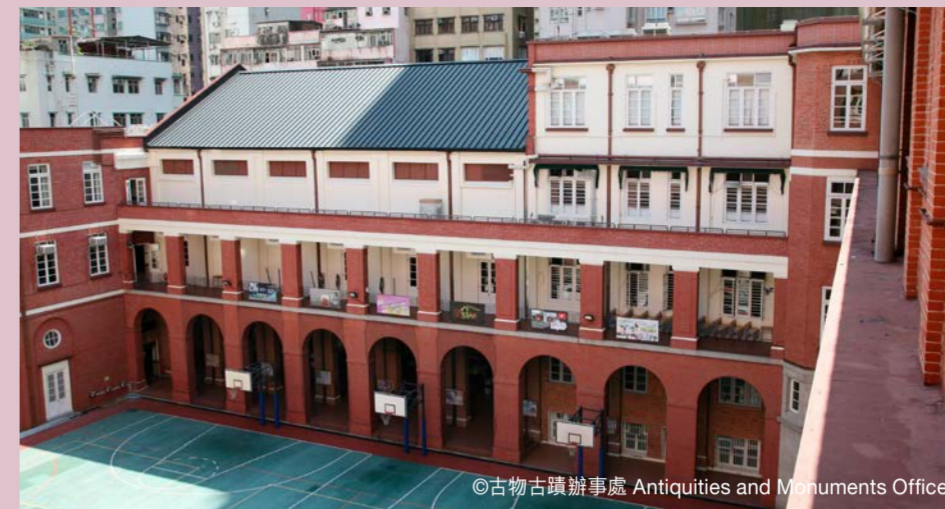
英皇書院的窗戶具古典風格的磚、石築砌緣飾，攝於2011年。 Windows of King's College are designed in the Neo-classical style with stone and bricks surrounds, 2011.
