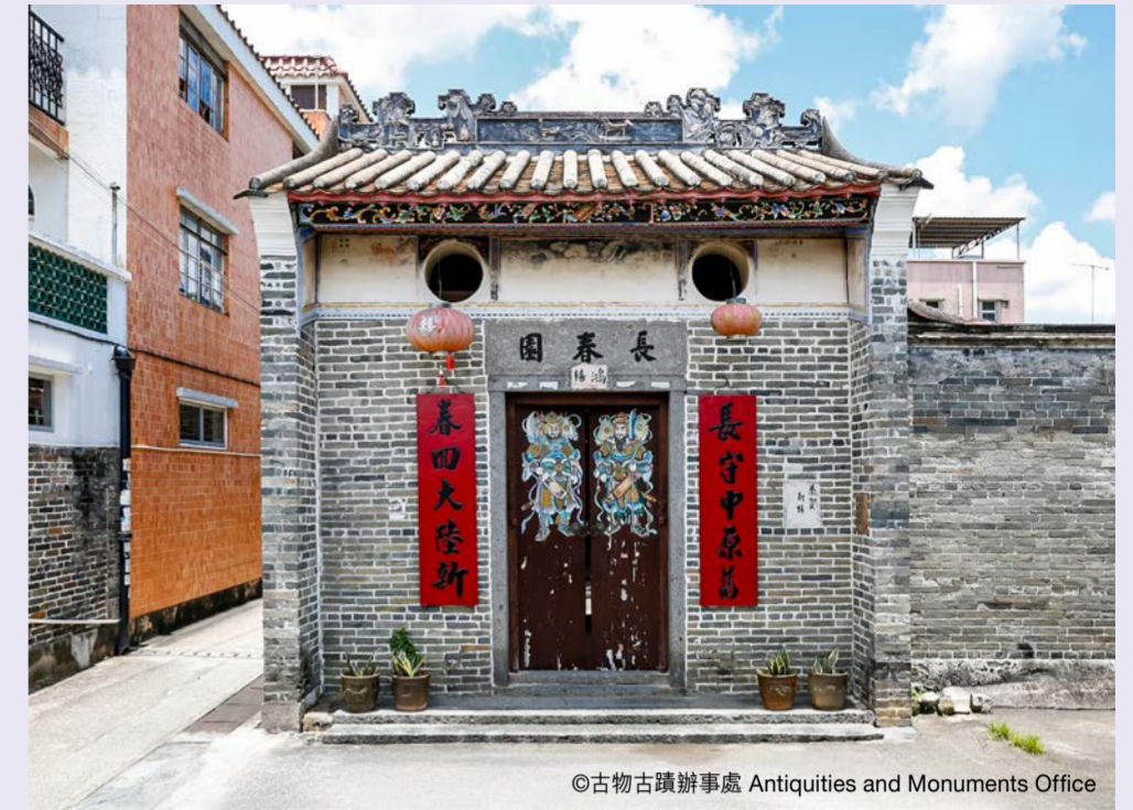
長春園正立面牆頭設有兩個圓洞，用作防禦，攝於2016年。 The two round openings on the wall frieze of the façade were for defence purpose, 2016.
